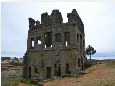
Figura 2 – Torre Centum Cellas
